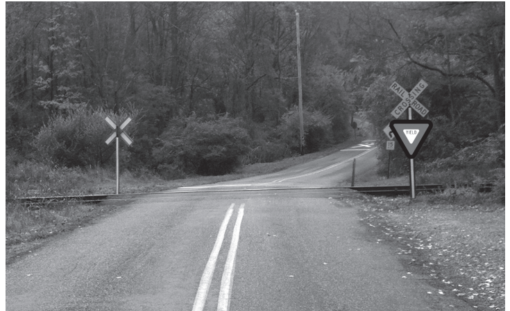
A YIELD or STOP sign must be installed at passive highway-rail grade crossings. In general, the rail company is responsible for installation and maintenance of these signs.
