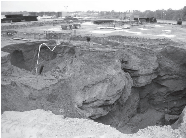
This large sinkhole opened up at a construction site.
